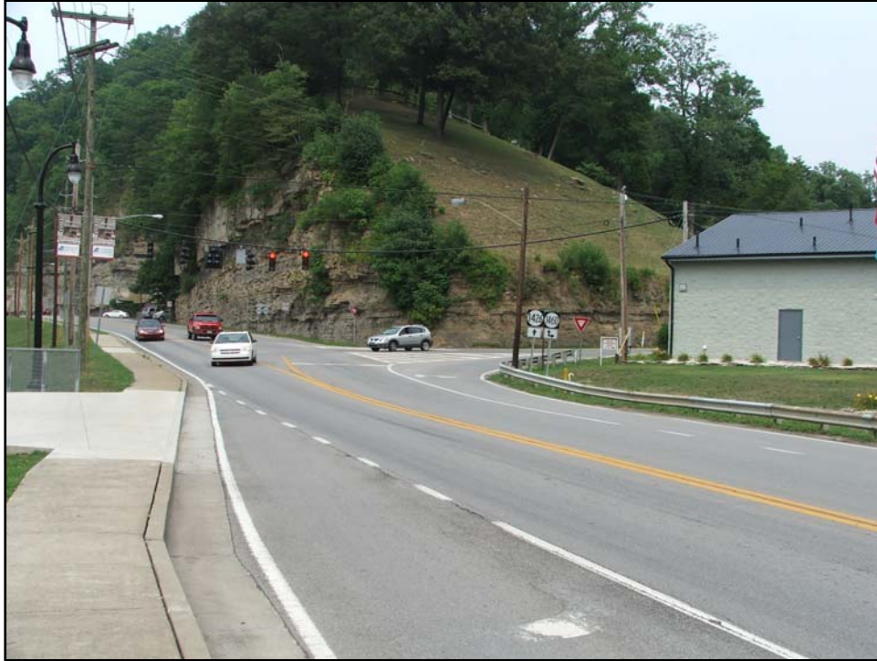
Cut slope at KY 1426/KY 1460 intersection with rockfall hazard. Dils Cemetery sits atop ridge
